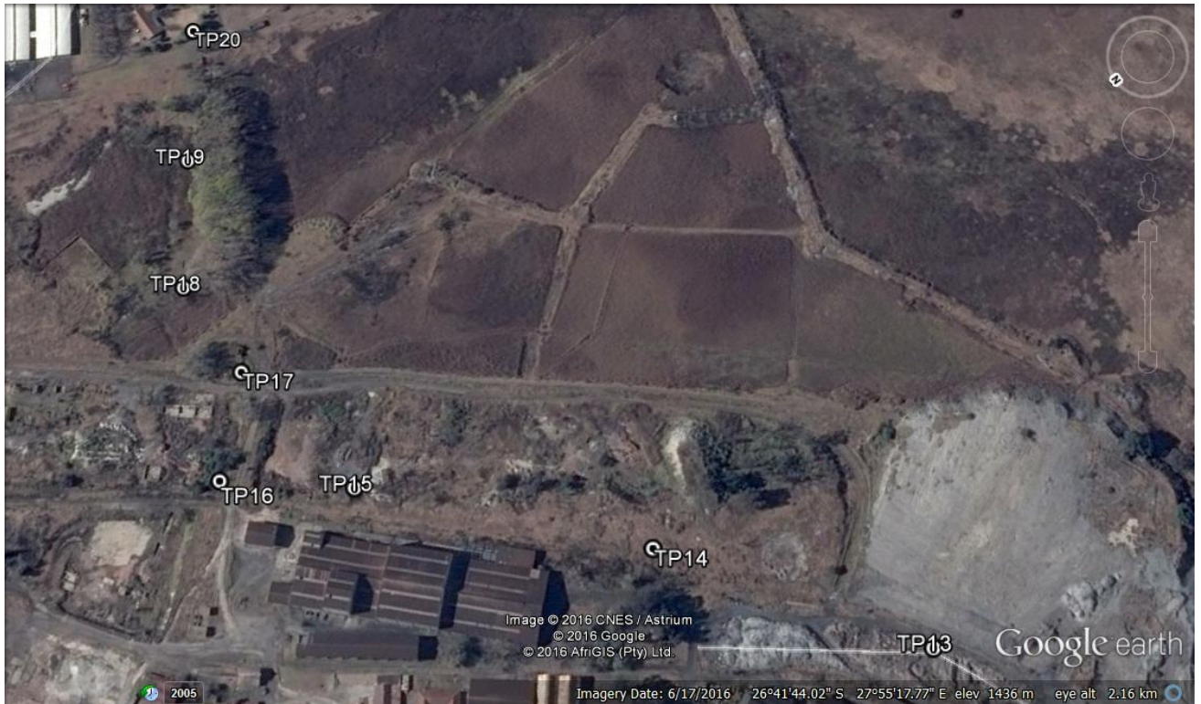
Figure 4: Water Logged Areas along the B19 Sludge Pipeline _ TP 13 to TP 20
